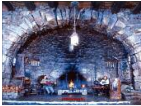
Great Fireplace at Hermits Rest Studio built by the Santa Fe Railroad in 1914.
